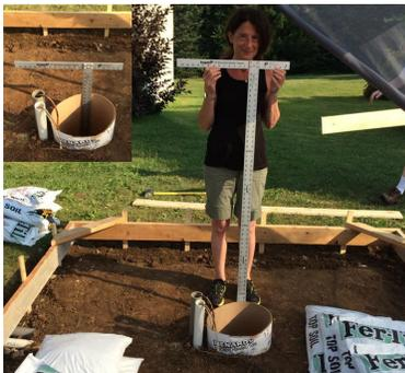
floor and pier. The hole for the isolated pier went down 40" deep. PVC pipes carrying communication cables were extended to reach the gap between the pier and the floor.
