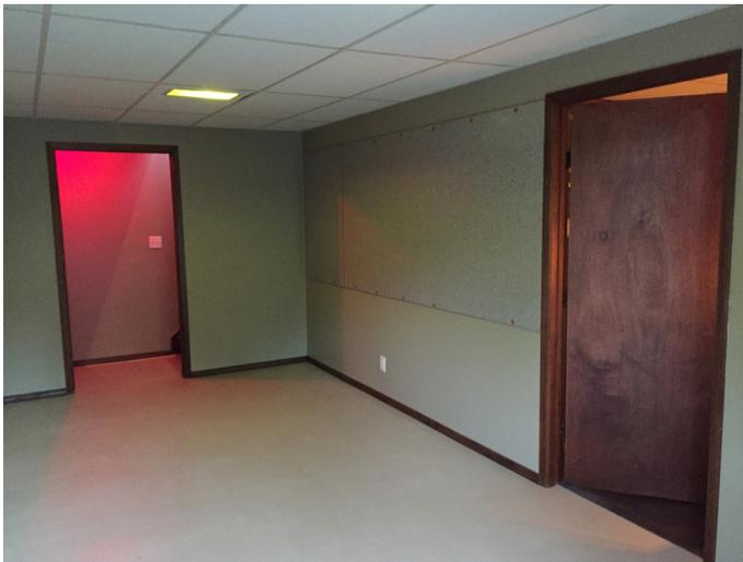
After transforming the old library-office space into a modern control room, we continued the remodeling of the Z-dome with the hallway. The ceiling tiles were refurbished, the walls were repaired and painted. The concrete floor was resurfaced with an epoxy paint. An addition of a trim molding made the floor work complete.
