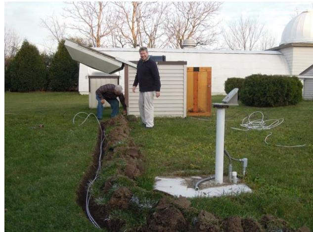
connections, we are using it with a pair of converters to give us a near 250 foot USB connection. The coax will be used to connect a camera so the telescope can be viewed from the control room.
