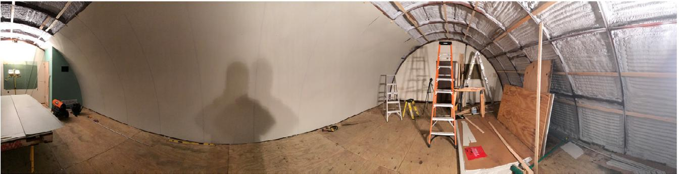
Great progress has been made on the Quonset remodeling project. During several well attended work parties one third of the new fiberglass-reinforced plastic wall panels were installed. The installation of different components of the electrical and audio-visual systems is underway. Everything has to be in
